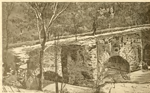
AQUEDUCT AT MISSION SAN JUAN.
